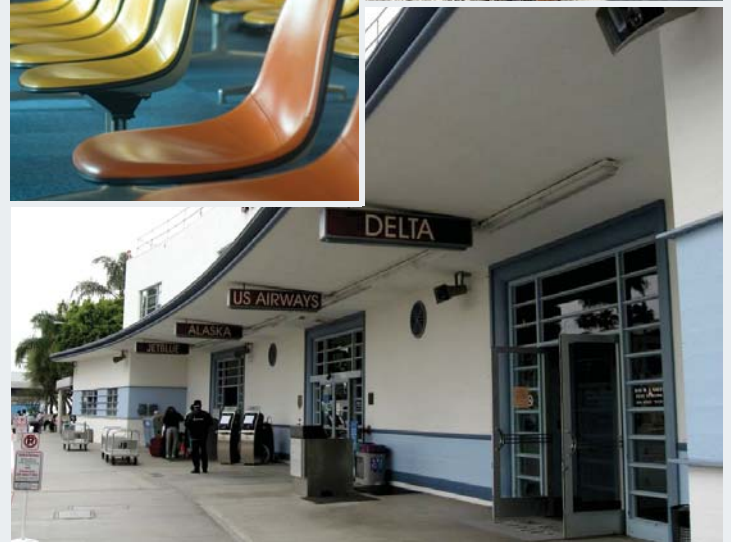
Airport facilities past their “useful lives”
